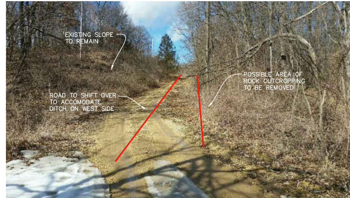
PICTURE OF ROAD LOOKING NORTH FROM STA 32+00
